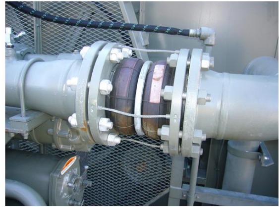
Figure 40: Rubber spherical pipe joint.
