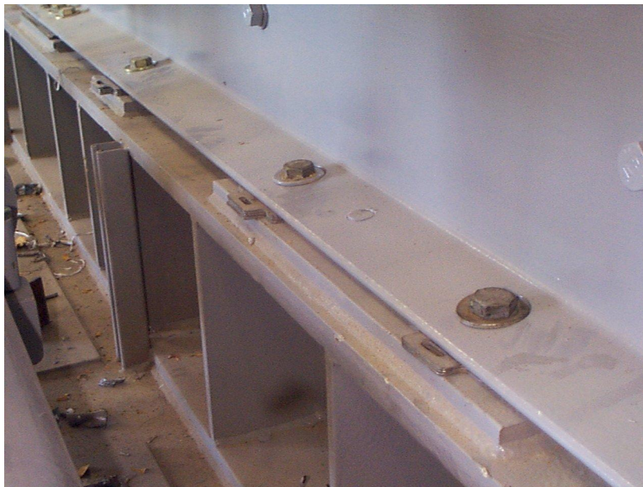
Figure 10: Example of mounting using shims.
