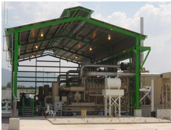
Figure 8: Example of compression package protected from the elements.
