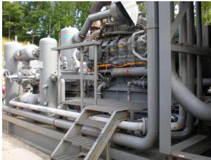
Figure 17: Work platform with staircase.
