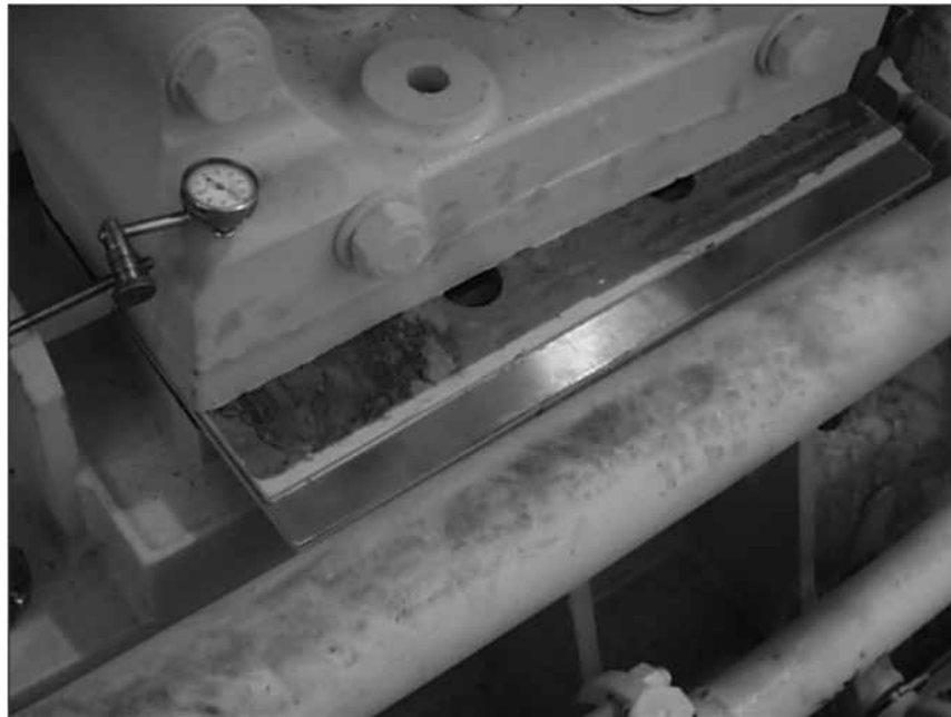
Figure 6.12 – Measuring Engine Soft-foot
