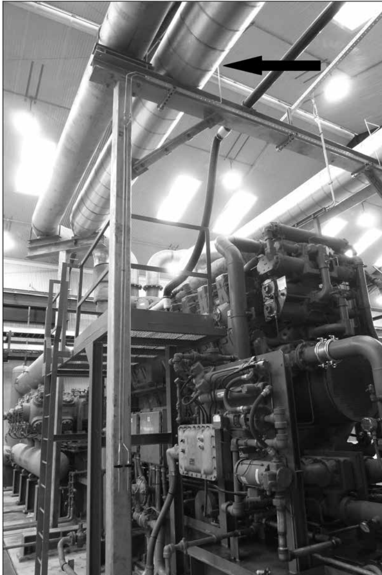
Figure 6.3 – Locate Emission Taps in the Straight Section or Exhaust Piping
