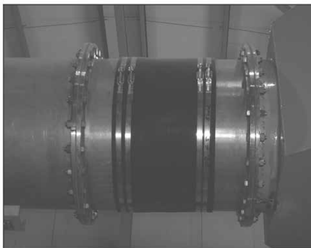
Figure 4.3 – A Good Example of Clamp Usage on Connecting Boots
