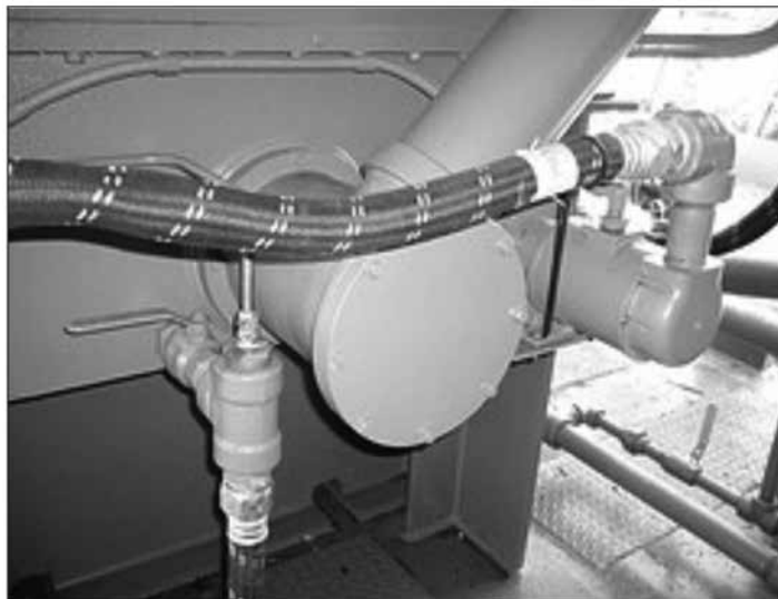
Figure 4.16 – Do Not Block This Oil Suction Screen Access Cover
